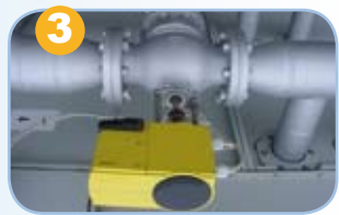
3 Modulating flow control valve (by-pass arrangement)
