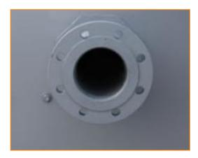
Flanges facilitate **piping connections** on-site.
