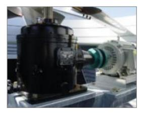
Gear drive system with close coupled motor
