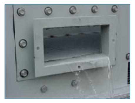
A factory-installed clean out port
