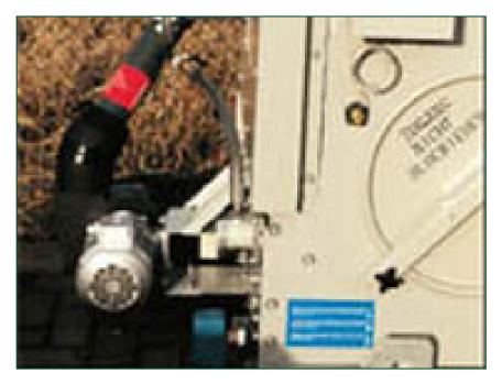
Relocate the water recirculation pump **at the connection end** for fans encased with sound attenuators and improve inspection and maintenance access.
