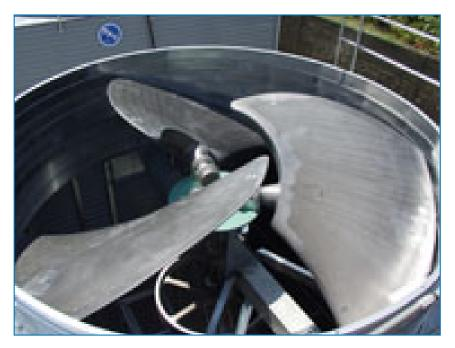
**Quiet and economical kW axial fans** mean S3000E cooling towers make little sound. To reduce noise still further, choose the **Whisper quiet fan** alternative targeting optimal noise-reduction, with an aluminum hinged-blade design and unique end caps.
