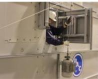
With the motor removal davit, the motor can easily be lowered from or lifted to the motor base without the need for extra heavy material of scaffolding.
