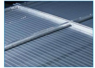
Dry finned discharge coil
