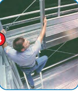
Internal ladder and service platform provides access to fan, motor, drives and coil.
