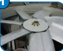
Low noise fans and full sound attenuation provide a total sound power level for the (4) condensers of 92 dB(A) which fully meets the requirement. At night-time the fan speed and noise level are further reduced to 85 dB(A) sound power level.
