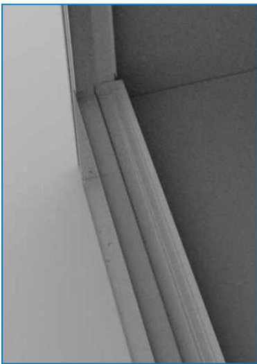
Water collection gutter
