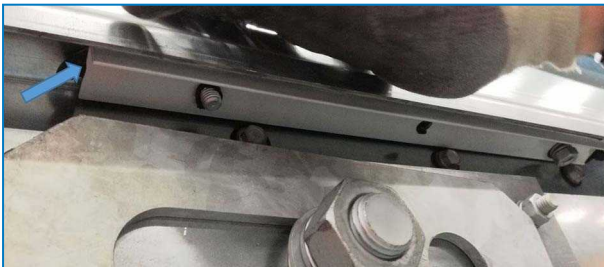
Installed sealing profile
