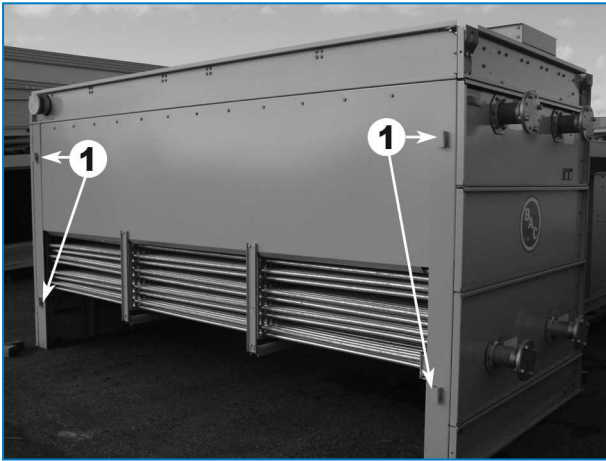
Male rigging guides on coil section
