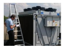
*Example:* Unit with 4 fans with 85 dB(A) in operation.
